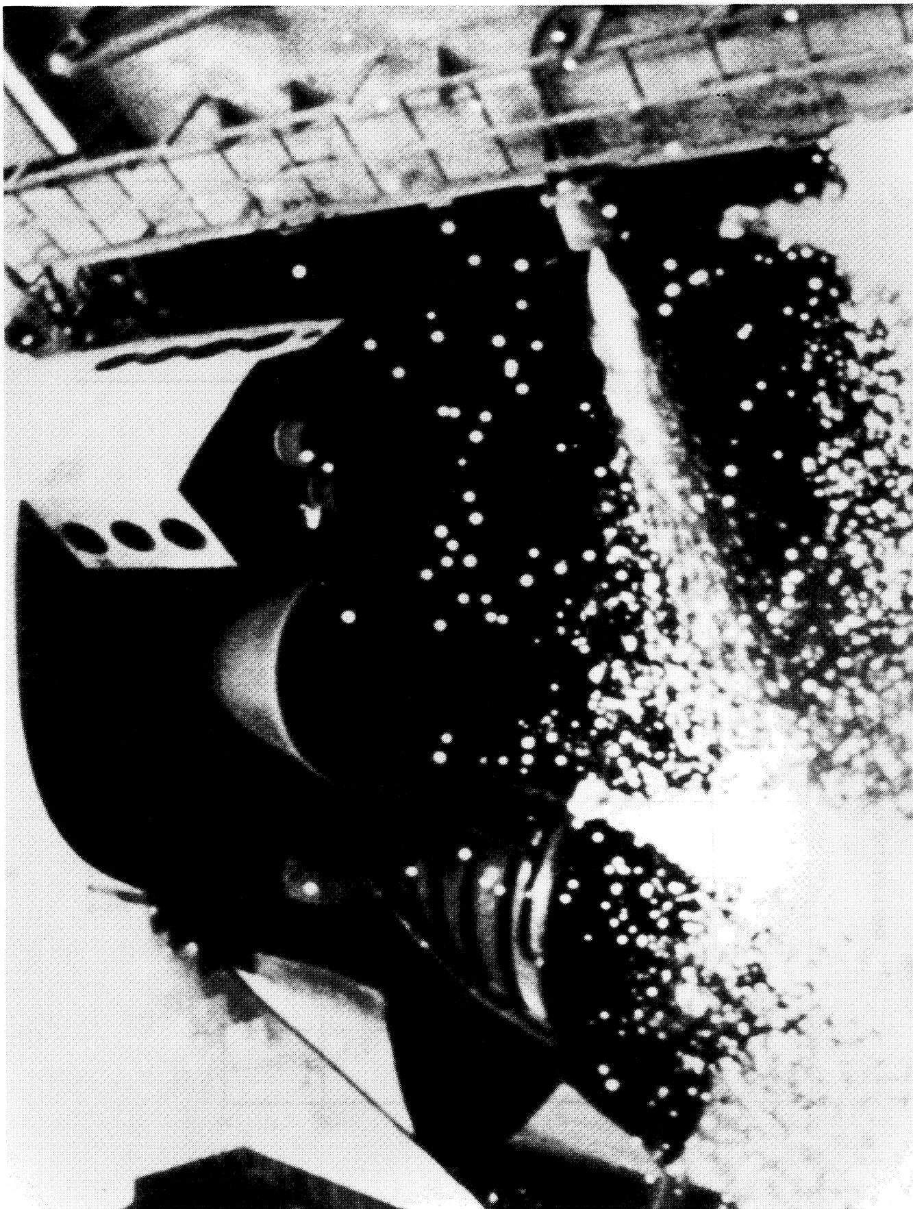
Figure 55. Radially outward firing initiator (ROFI) located on KSC's LC-39.
