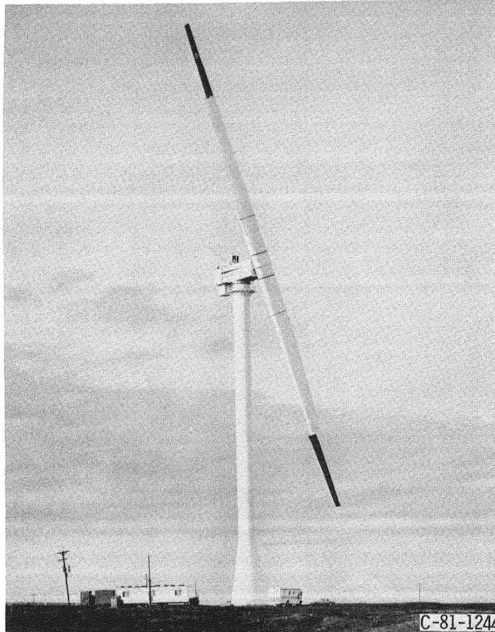
Figure 3. - Mod-2, 2.5 megawatt wind turbine. Tower is a steel circular cylinder on a steel conic base.
