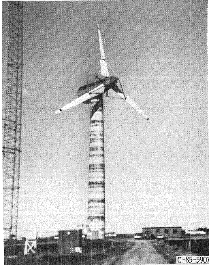
Figure 4. - Nibe A, 630 kW wind turbine. Tower is constructed of reinforced concrete by slip forming.
