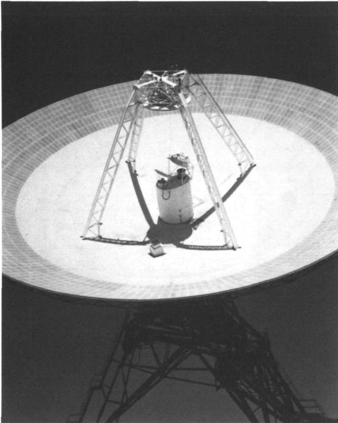
Fig. 1. DSS 12 34-m HA-Dec antenna with S/X reflex feed system
