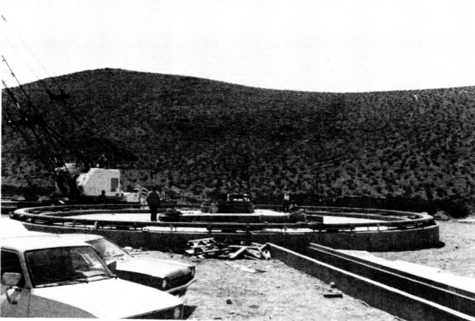
Fig. 6. Track and support runner, DSS 15
