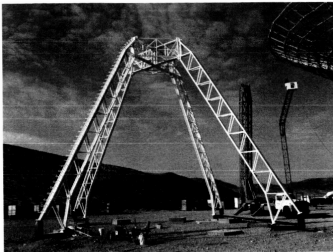
Fig. 13. Quadripod structure, DSS 15
