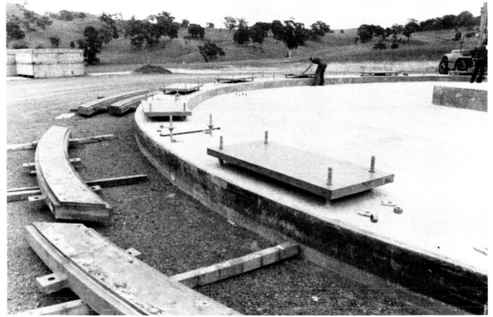
Fig. 3. Track foundation and runner support
