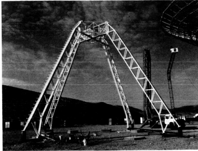
Fig. 13. Quadripod structure, DSS 15
