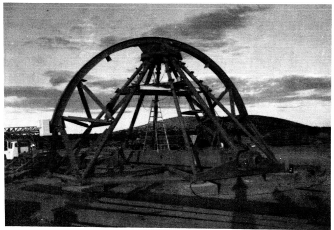
Fig. 8. Tipping structure support and elevation bearing
