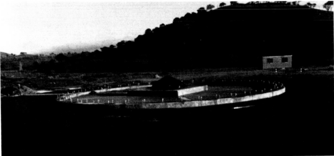
Fig. 2. Foundation, 34-m Az—El antenna, DSS 45
