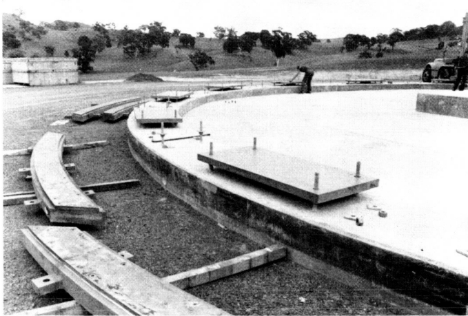
Fig. 3. Track foundation and runner support
