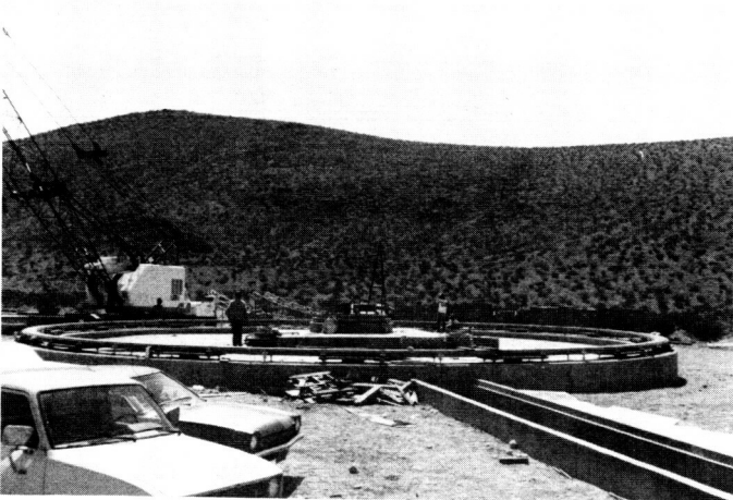
Fig. 6. Track and support runner, DSS 15
