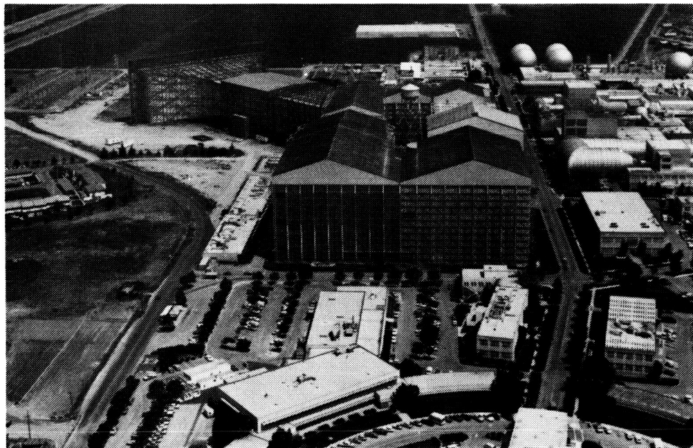
(b) Looking at south wall of the 40 \times 80 tunnel.
