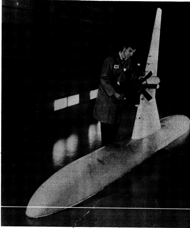
FIGURE 1. STRAIGHT UNDERWING NACELLE MODEL IN AMES TUNNEL
