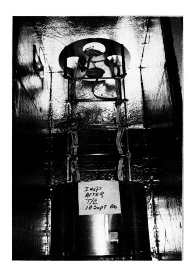
Figure 9: Boom Deployed in Thermal Chamber
