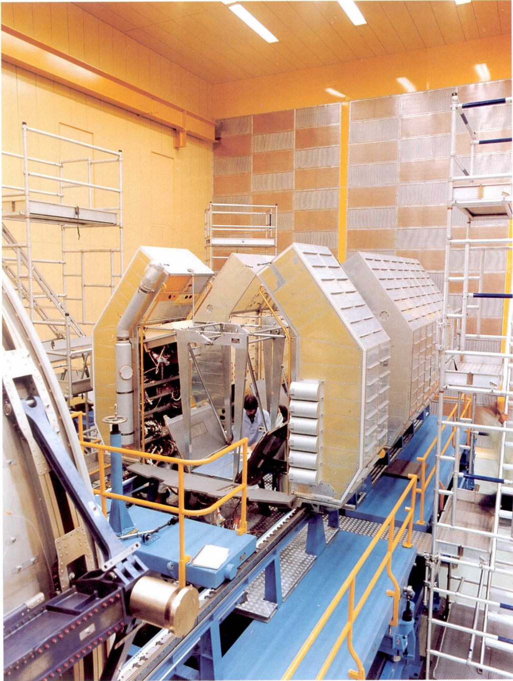
Figure 71. Preparation and installation of subsystems and racks for engineering model test T 006 at ERNO in October 1978.
