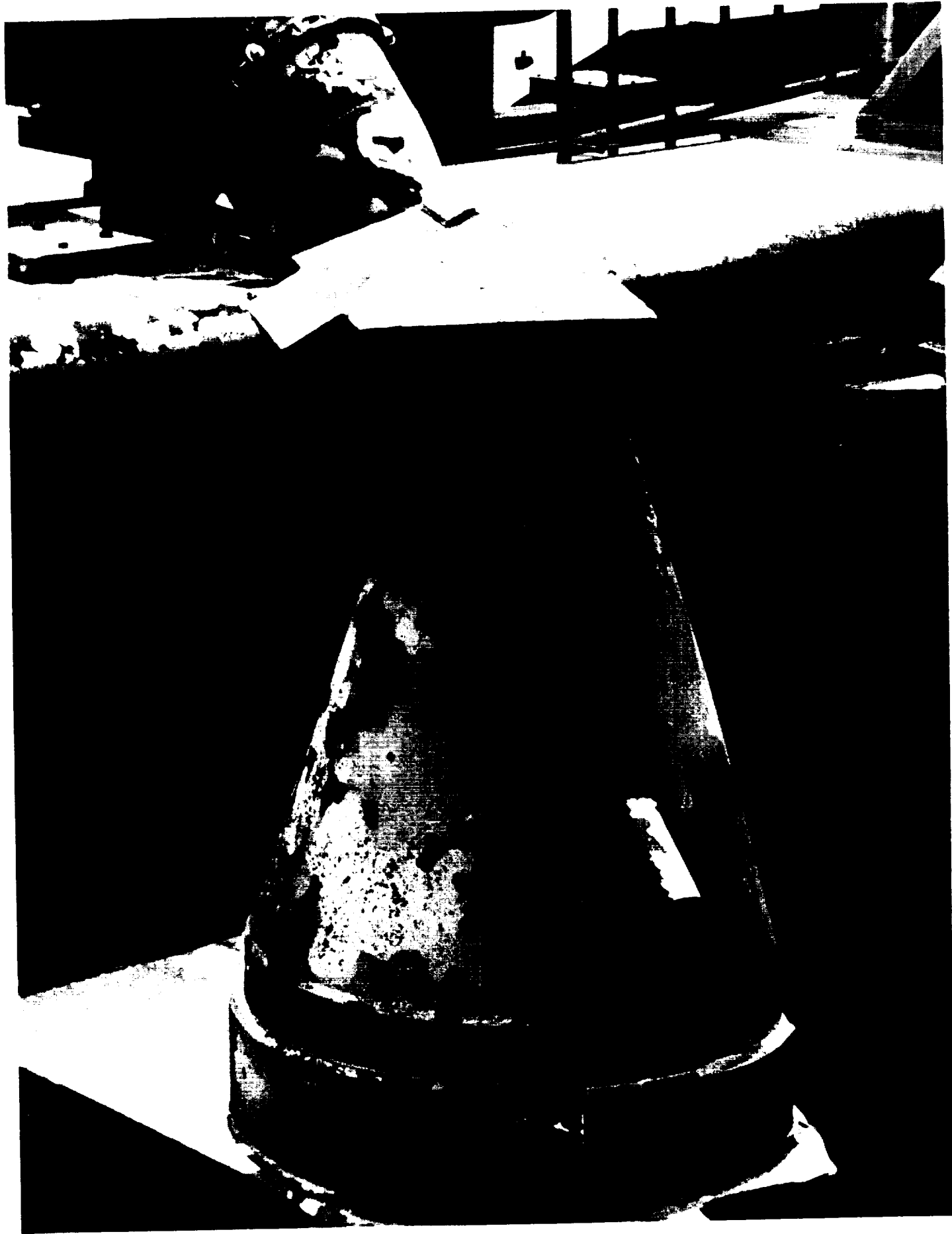
NORTH HOLDDOWN POSTS SUSTAINED NEGLIGIBLE EROSION. DOGHOUSE BLAST COVERS HAD CLOSED PROPERLY
