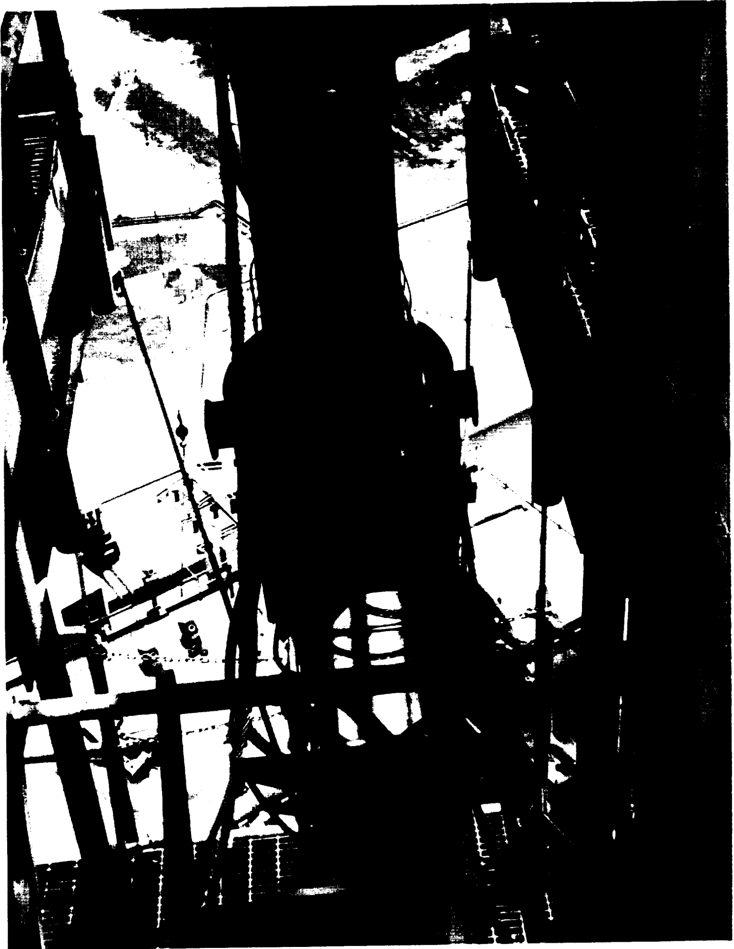
GH2 VENT ARM LATCHED, BUT WAS CAPTURED 'OFF-CENTER'
