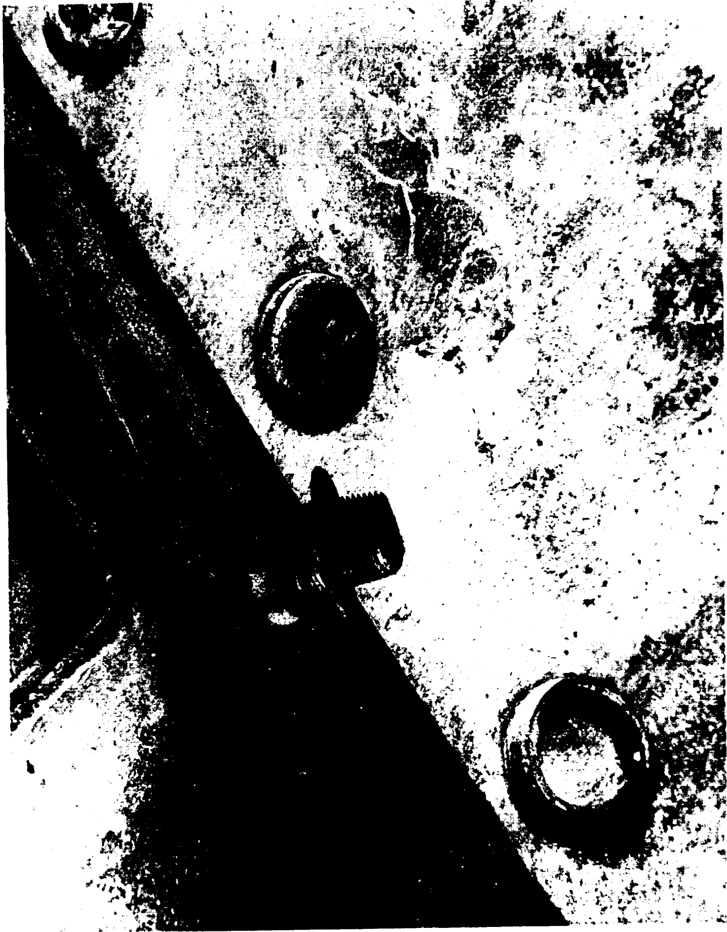
LOOSE BOLT IN A MOBILE LAUNCH PLATFORM ACCESS COVER
