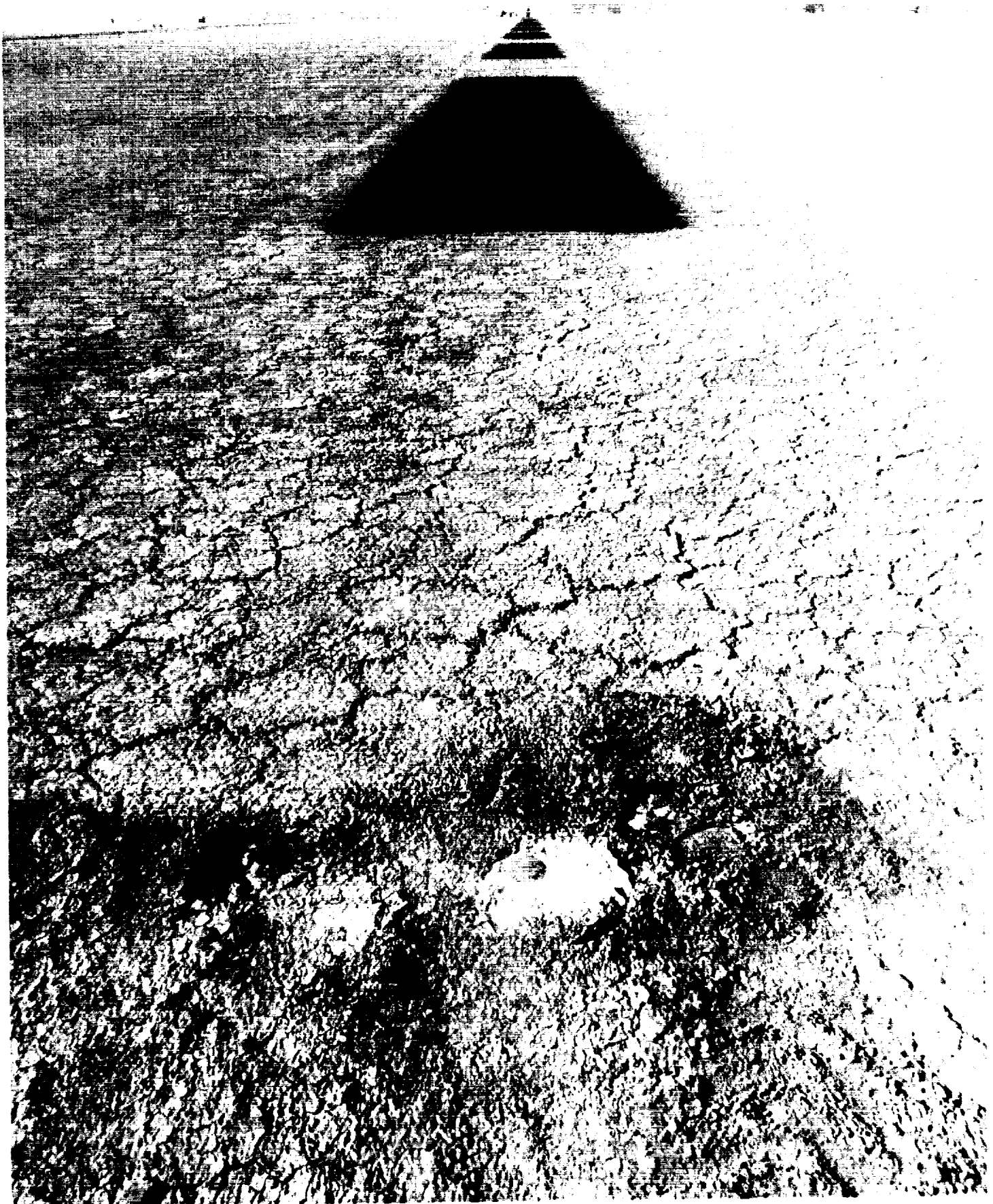
Survey marker/concrete post protruded 3/4-inch above Runway 23 surface 287 feet away from the Orbiter touchdown point
