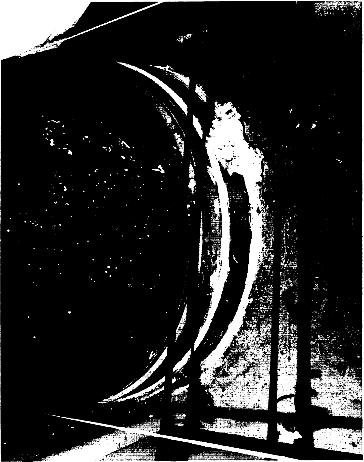
Excessive application of RTV to the SRB holddown posts
