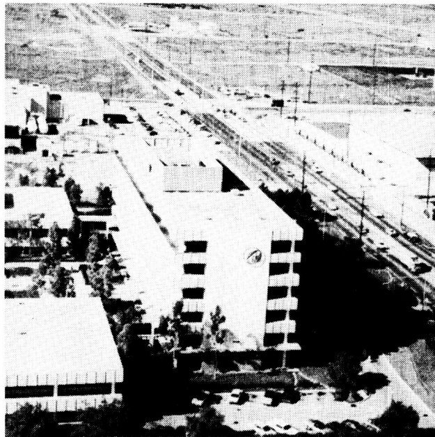
Figure 8d. Building at 1.5 BPP.
