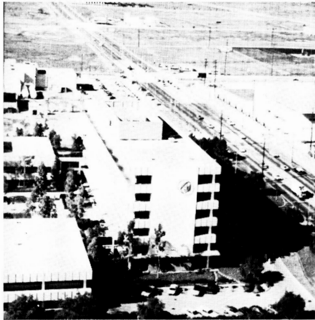
Figure 8b. Building at 2.4 BPP.
