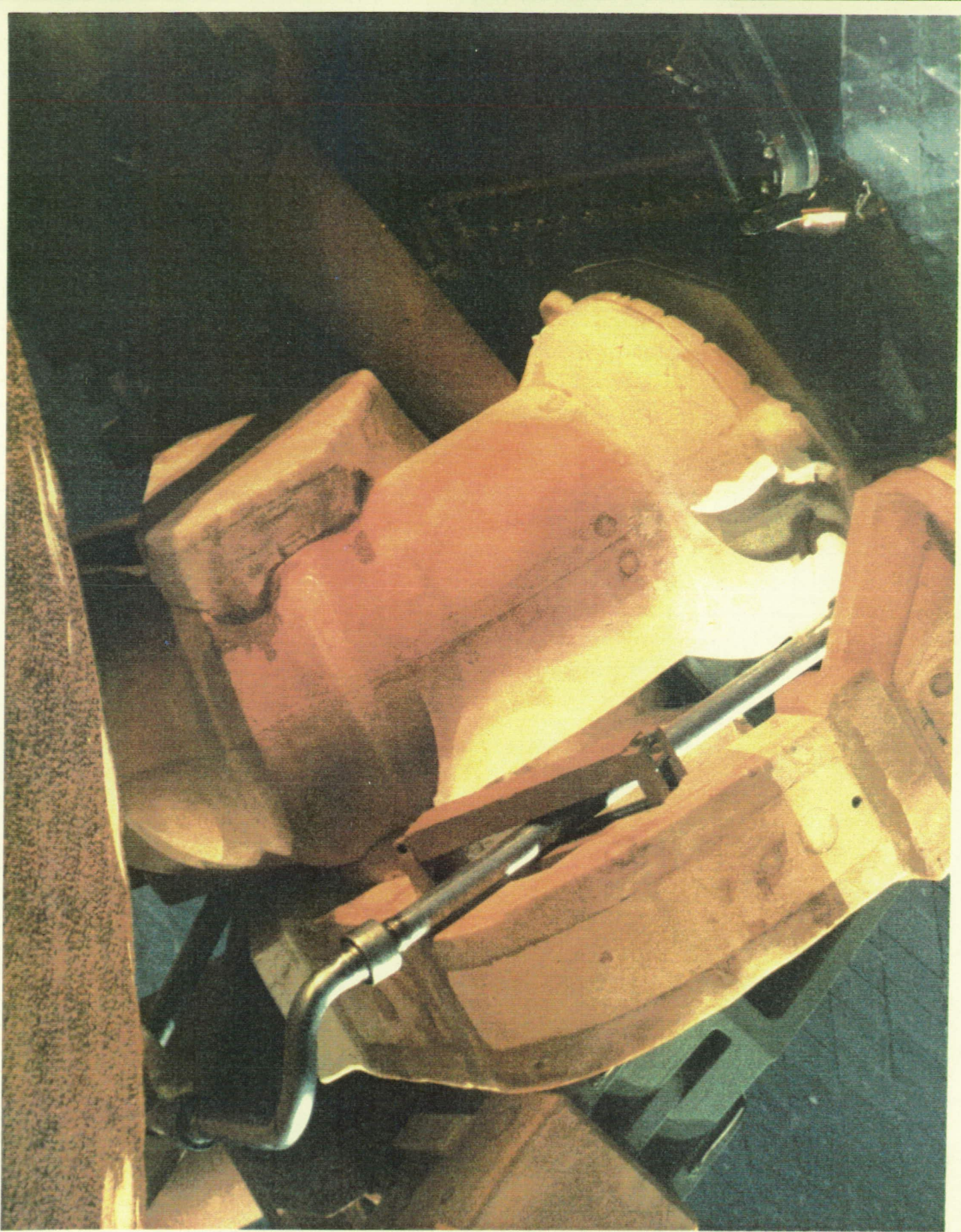
Ice/frost accumulation on the LO2 ET/ORB umbilical occurred on the aft and inboard sides, and on the purge vents
