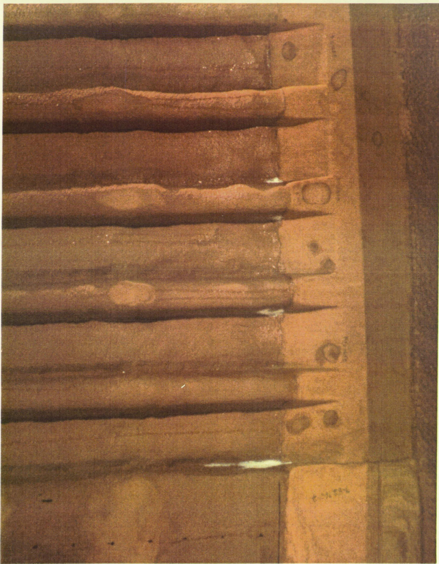
Frost accumulations in the intertank stringer valleys occurred on the -Z side of the tank
