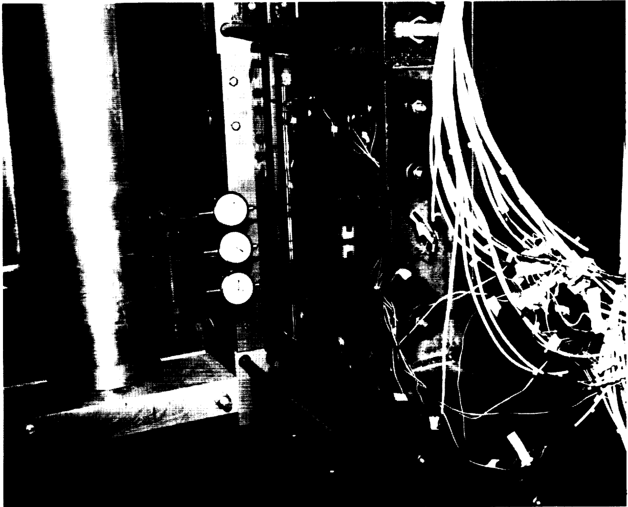
FIGURE 119. CLOSE-UP OF DIAL INDICATORS ON THE TITANIUM SIDE OF THE LARGE SLIDING-JOINT PANELS — ROOM TEMPERATURE CONDITION
