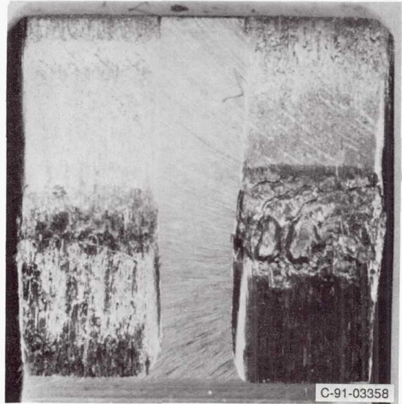
(a) Typical fatigue spall.
