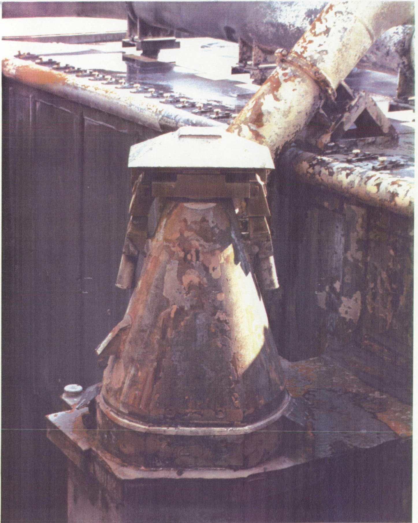
All doghouse blast covers on the north holddown posts had closed properly. Plume erosion appeared to be less than usual.
