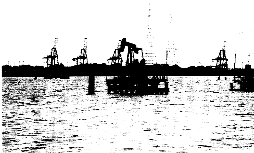
FIGURE 3-8. Submerged oil wells in the Goose Creek Oil Field near Baytown, Texas. These wells were once located on dry ground until subsidence in the oil field left them in their current, partially-submerged state.
