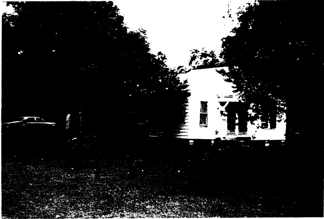
FIGURE 3-3. Residence that straddles the Wooster fault in Baytown.
