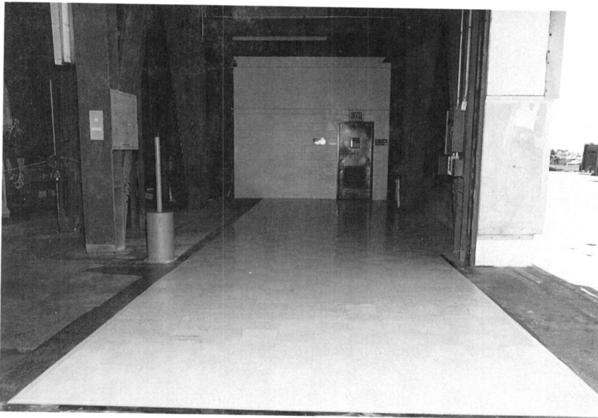
Floors at the Vehicle Assembly Building in the Low Bay
