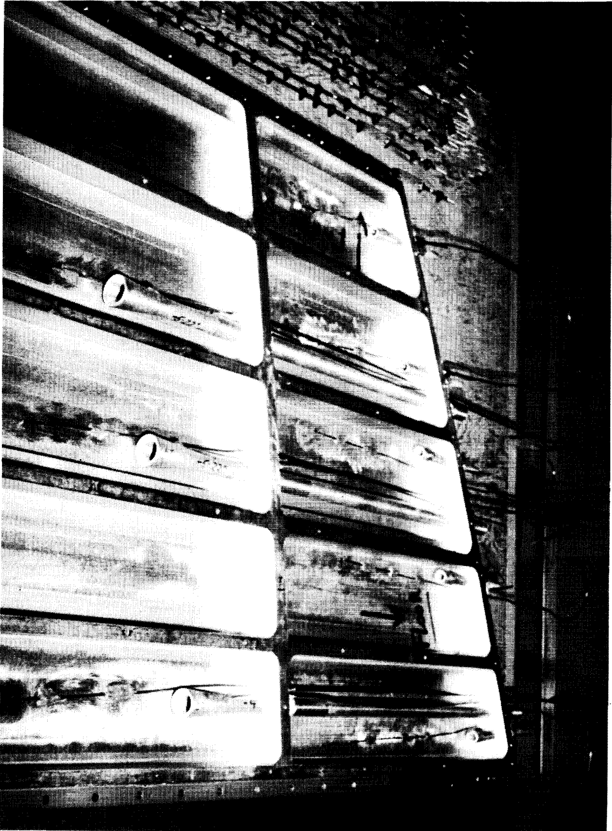
(b) Photograph of nozzles in ducts. Figure 15. Concluded.
