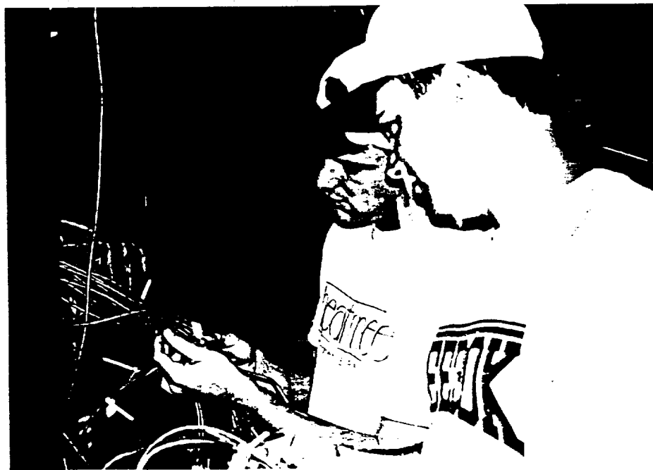
SORTING STRAIN GAUGE LEADS
