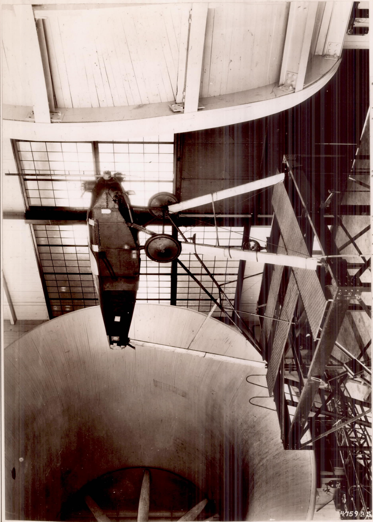
Fig. 1 Sperry Messenger fuselage mounted in the propeller research tunnel
