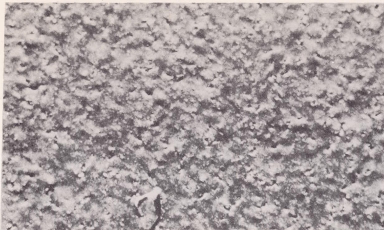
(a) Condition of coating before tubercules had begun to form. Note discontinuities in the coating (probably caused largely by gas evolution from the metal during the firing process).
