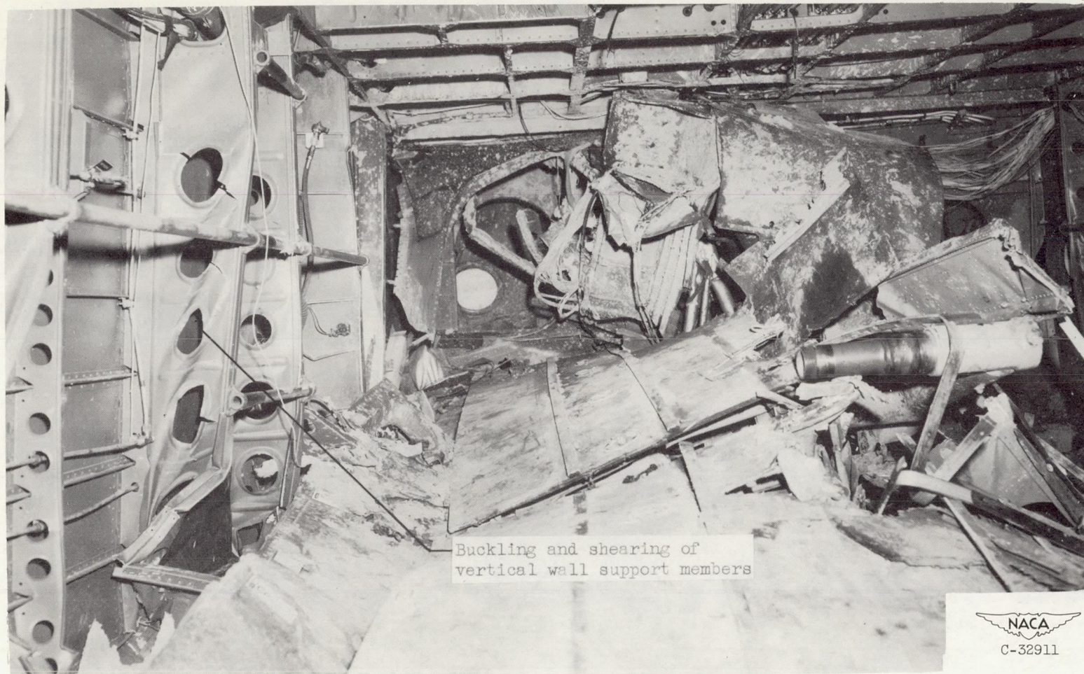
(b) Buckling and shearing of vertical wall members.
