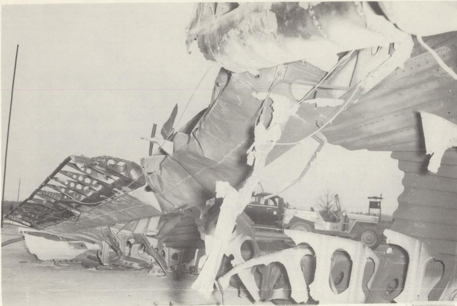
(b) Rear view of damage to wing structure.
