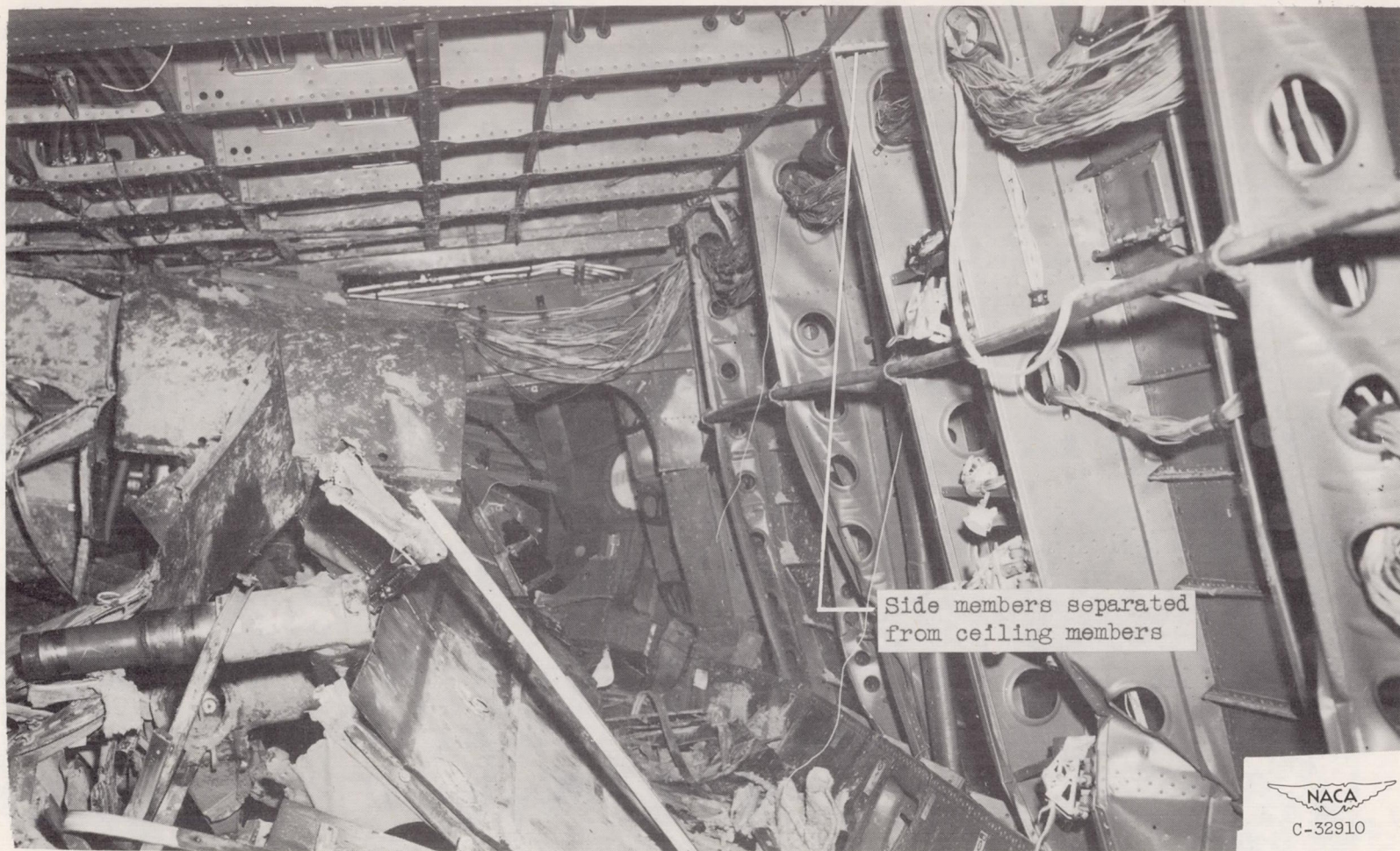
(a) Side members separated from ceiling members.
