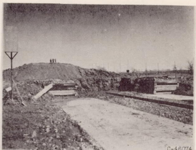
(a) Earth and timber abutments that ripped landing gear from airplane upon crash.
