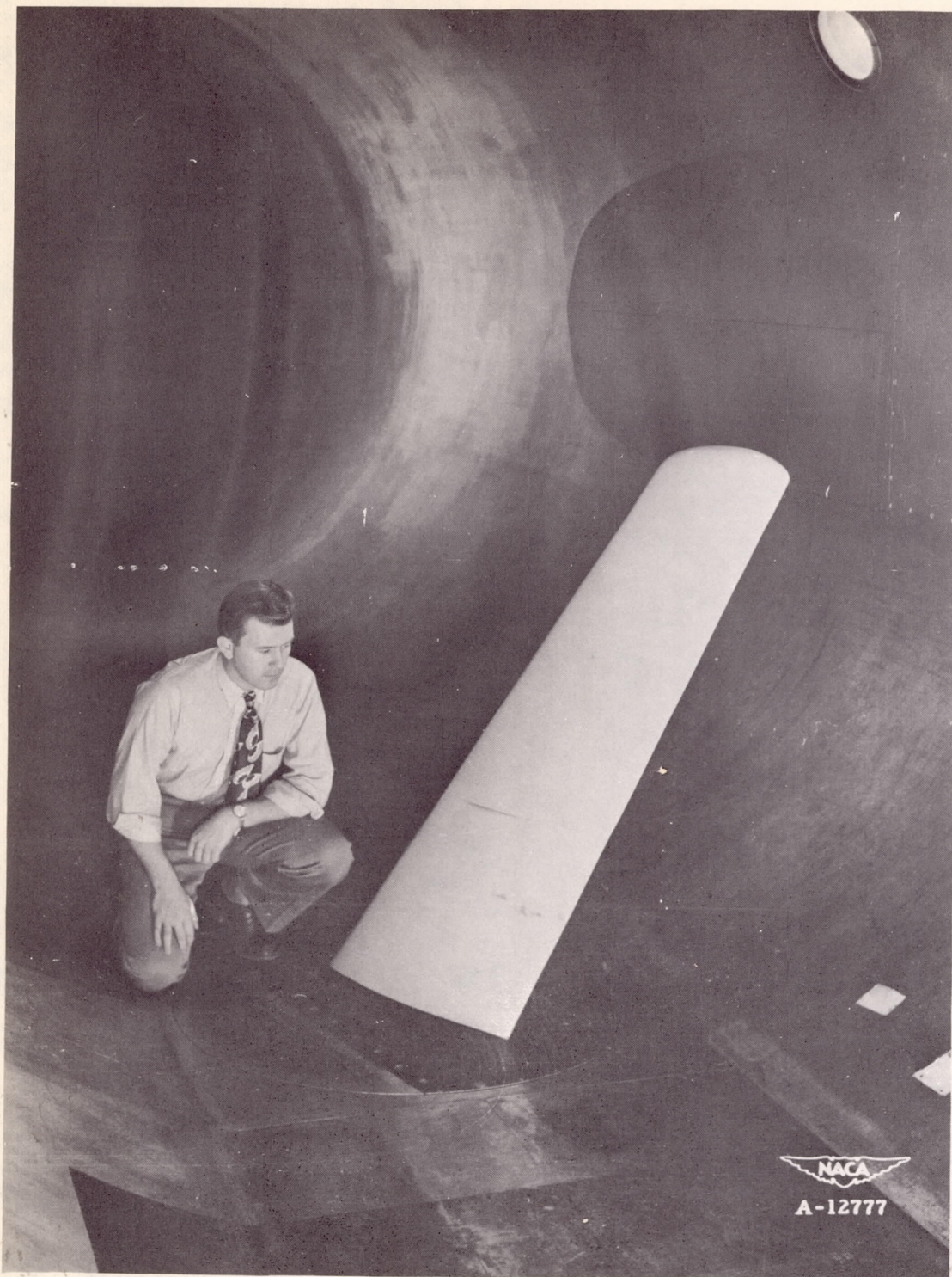
Figure 5.- Semispan wing mounted in the Ames 12-foot pressure wind tunnel.
