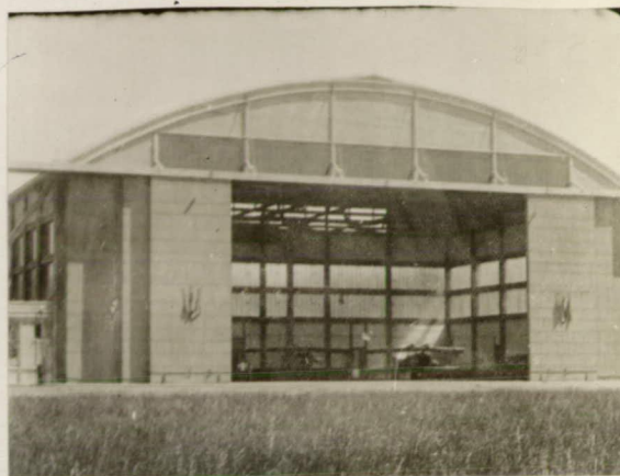
Reinforced concrete hangars at Le Bourget, with electrically operated doors. Their tremendous height may be judged from the Spau 46 and Farman Goliath planes which are visible within.
