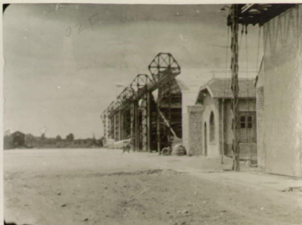
Hangar installation at headquarters of Latecoere Line, Toulouse, France.
