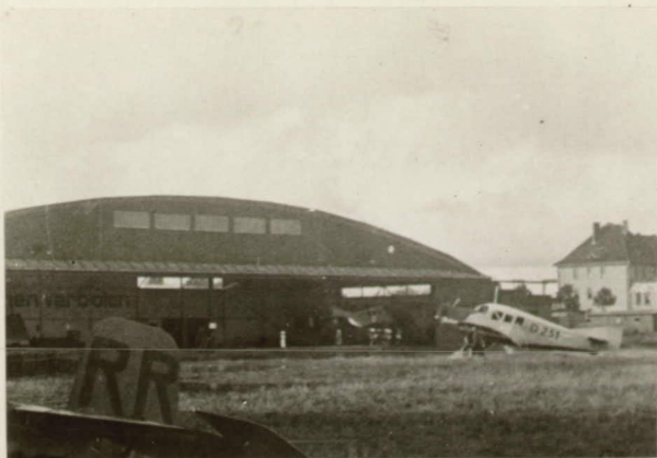
Municipal hangar and Customs building at Königsberg, East Prussia.
