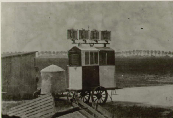
Flood light installation at Le Bourget. Arklight under hood; motor-generator set in shack
