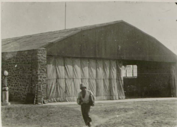
Latecoere installation at Rabat and Casablanca, Morocco.
