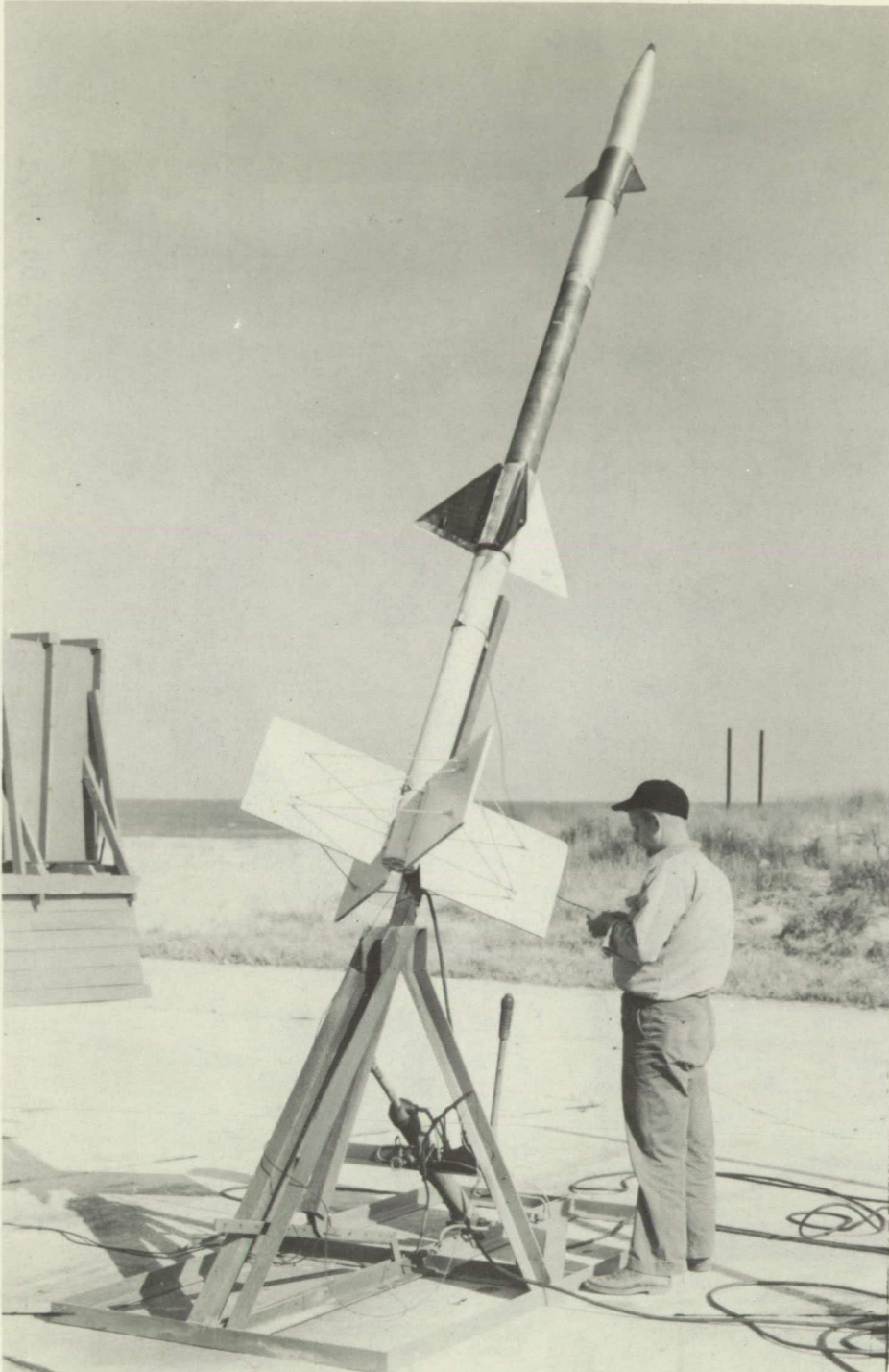
(b) Vane-spoiler configuration with booster on launching stand (model 6).
