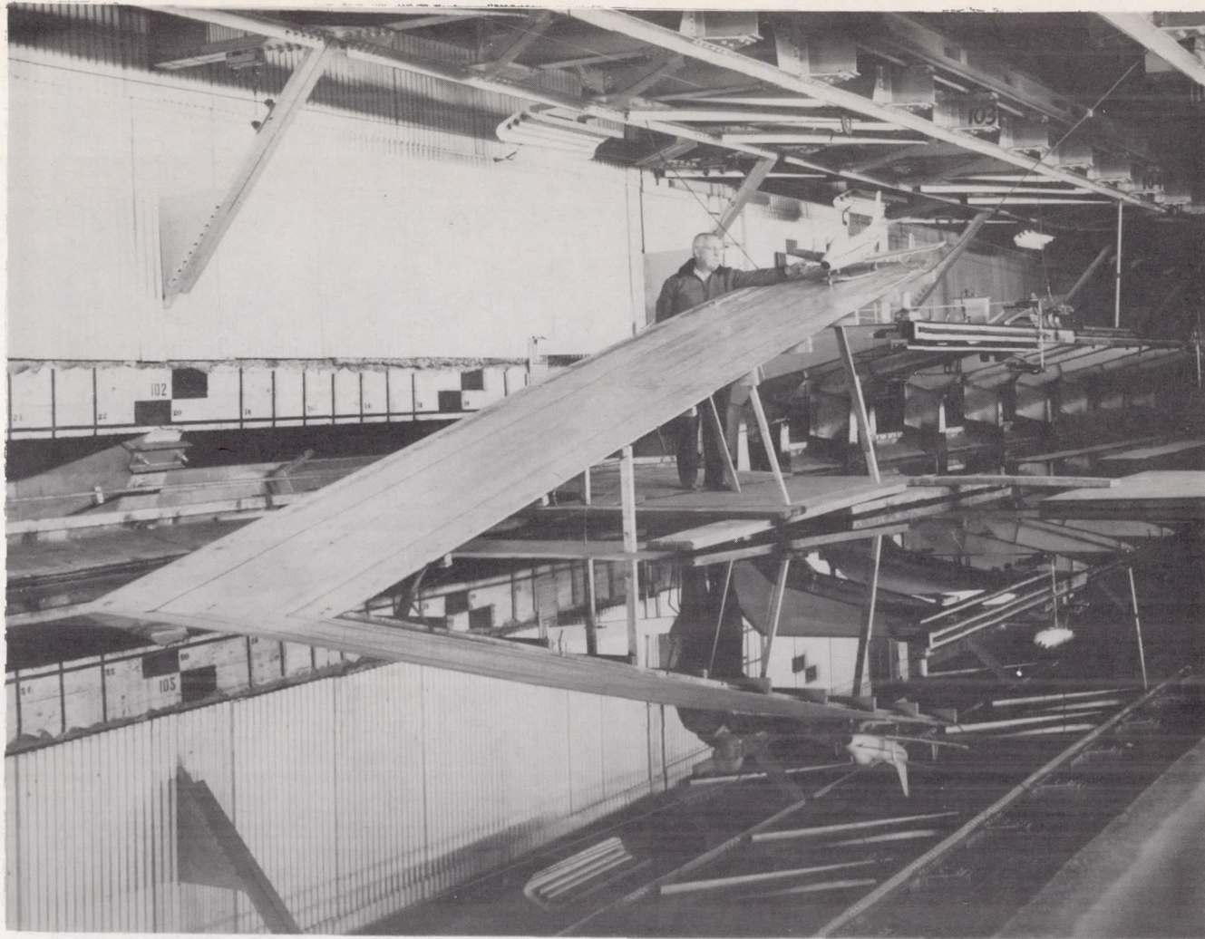
L-93380 Figure 5.- Ramp setup for ramp-to-water transition in Langley tank no. 2.
