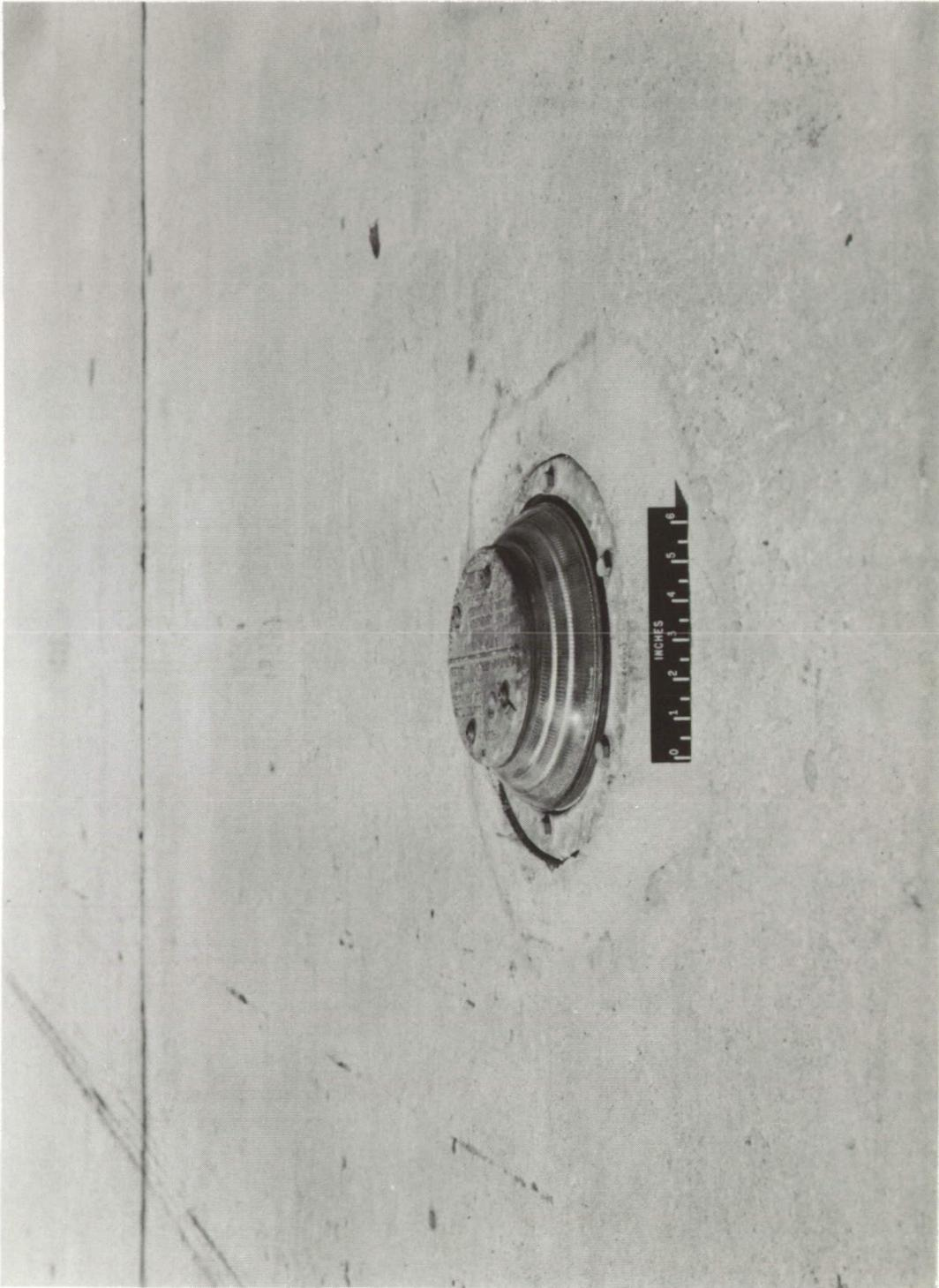
Figure 5.- ANL-9 light installed in runway at Langley landing-loads track. L-57-4068
