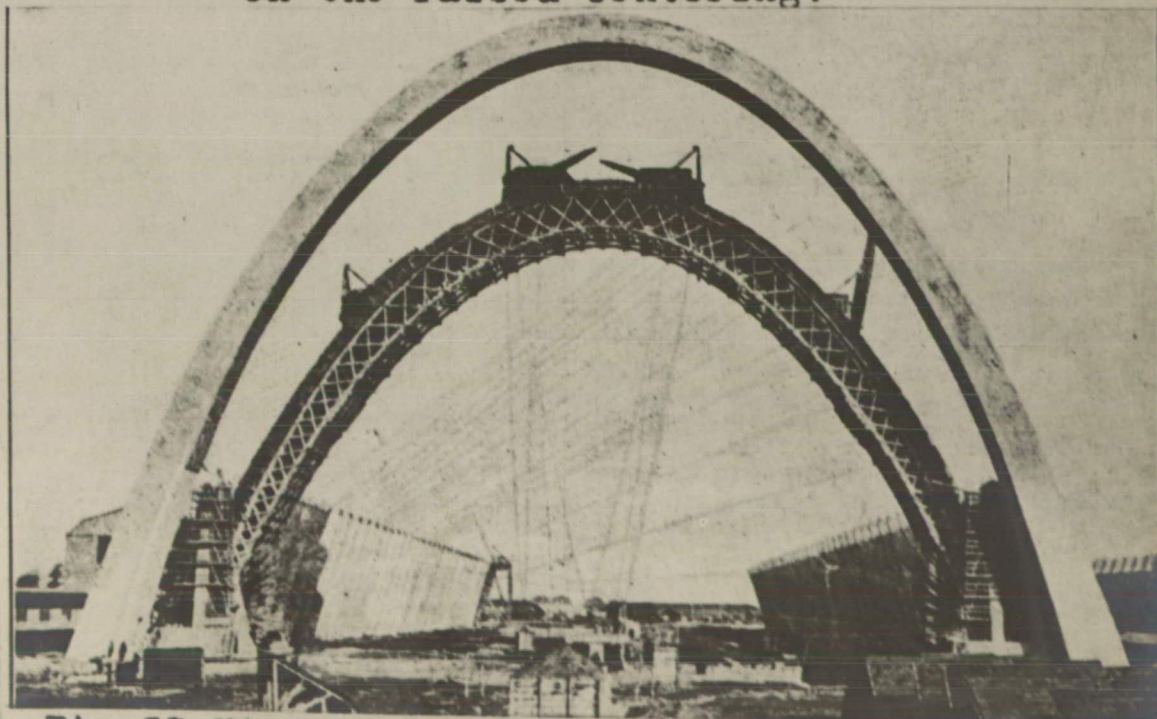
Fig. 37 View of finished arch and of centering lowered for shifting.
