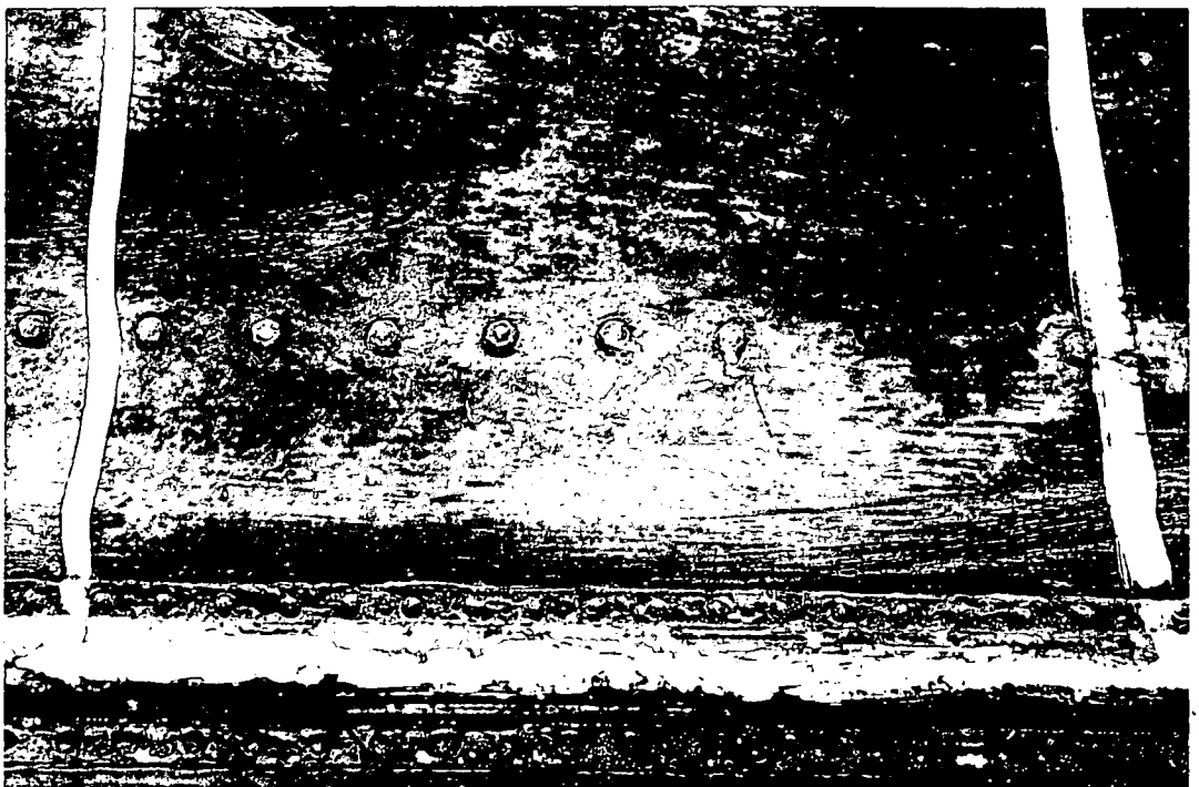
Fig.2 Note corrosion of rivets due to lack of protection afforded by an anti-corrosive anti-fouling paint.
