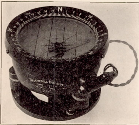
FIG. 10.—Campbell-Bennett aperiodic compass, Type 6/18, Mark II.
