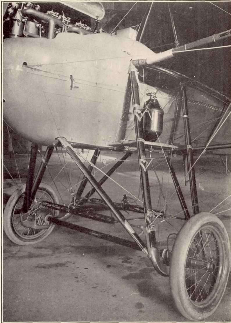
Fig. 27.—Tensiometer attached to wires.
