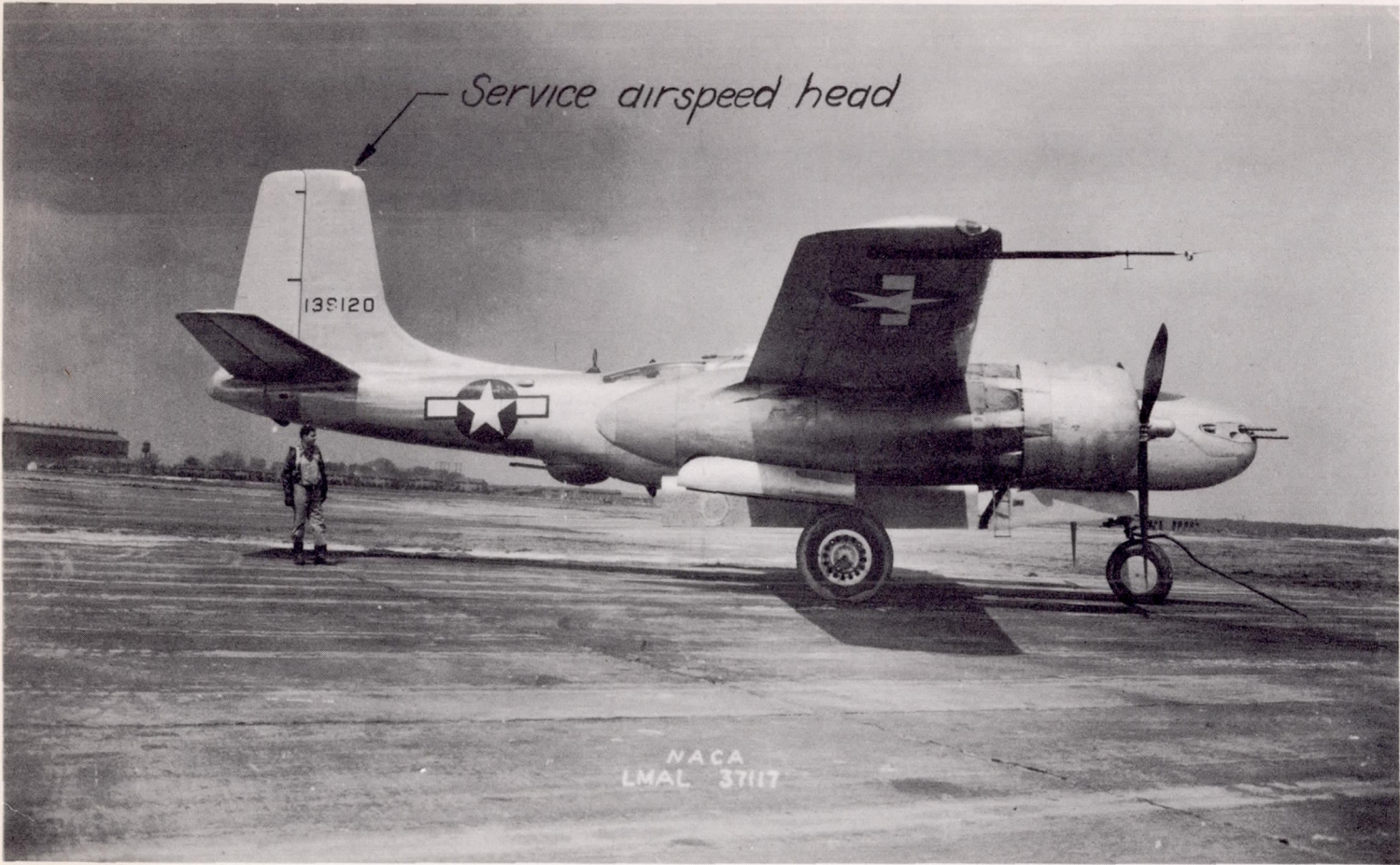
Figure 3.- Side view of Douglas A-26B airplane showing service airspeed head.
