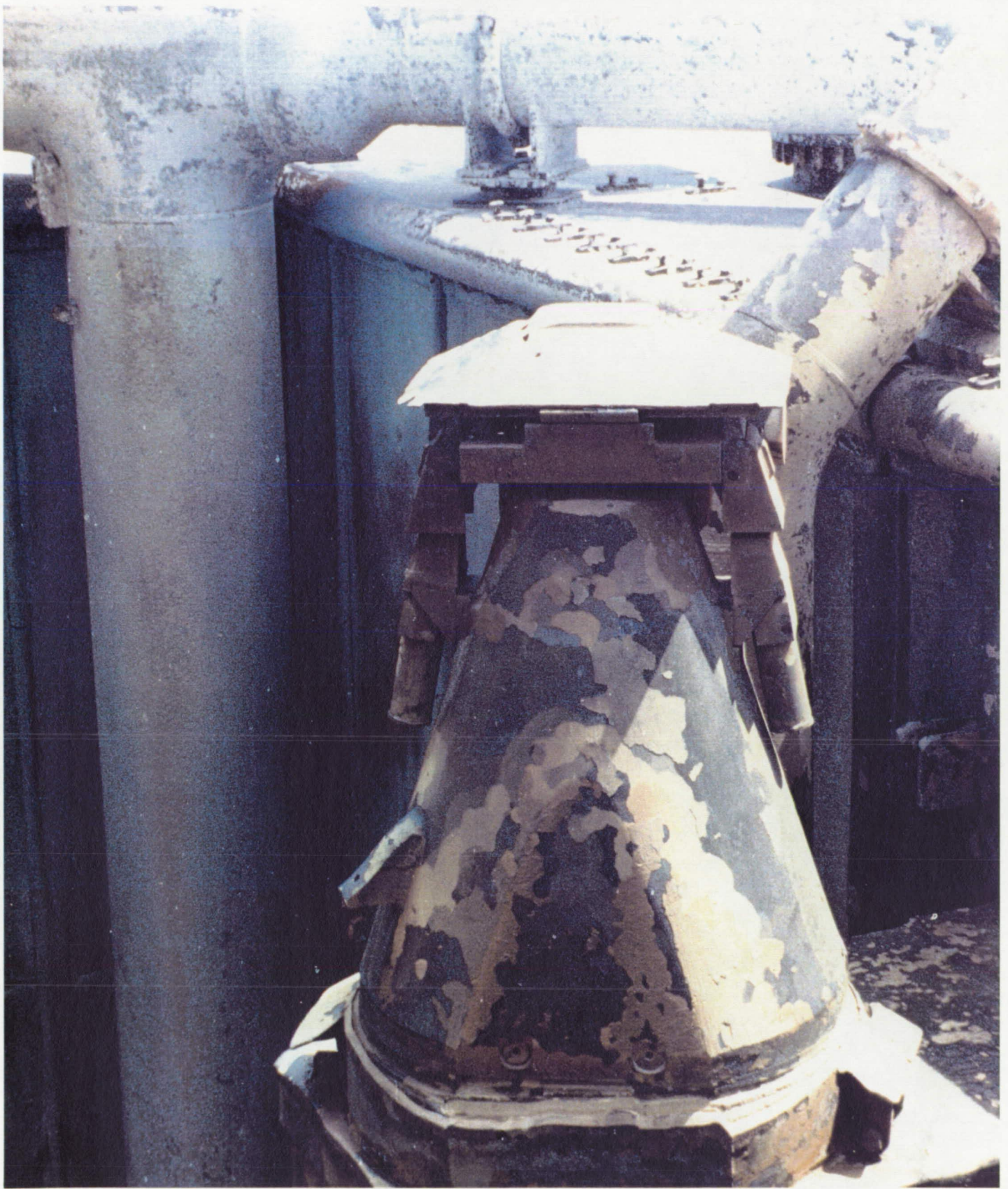
SRB plume erosion of the north HDP blast covers was typical with the exception of the HDP #4 cover, which had several burn-through holes.
