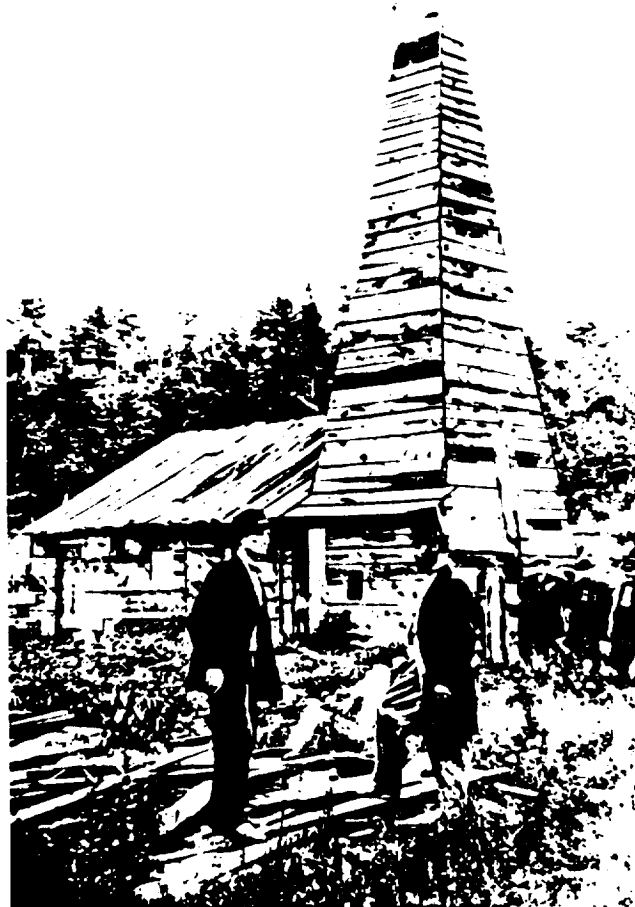
The derrick used in the drilling of oil wells, such as Drake's, was exactly the same as had previously been used for brine.
