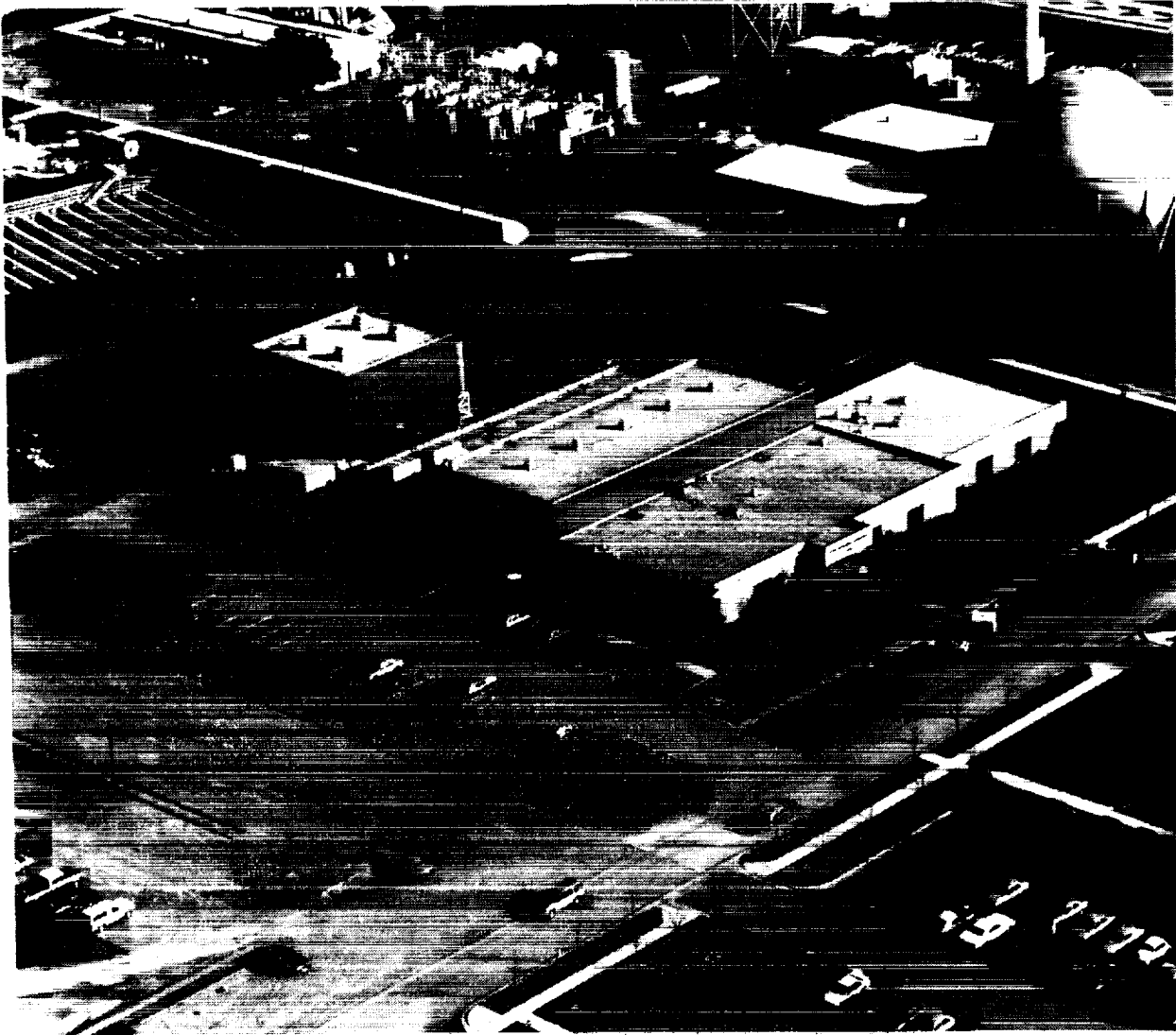
Aerial view of the NASA Ames Fluid Mechanics Laboratory. Front to back: office wing, stand-alone wind tunnels, indraft wind tunnels, and compressor building.
