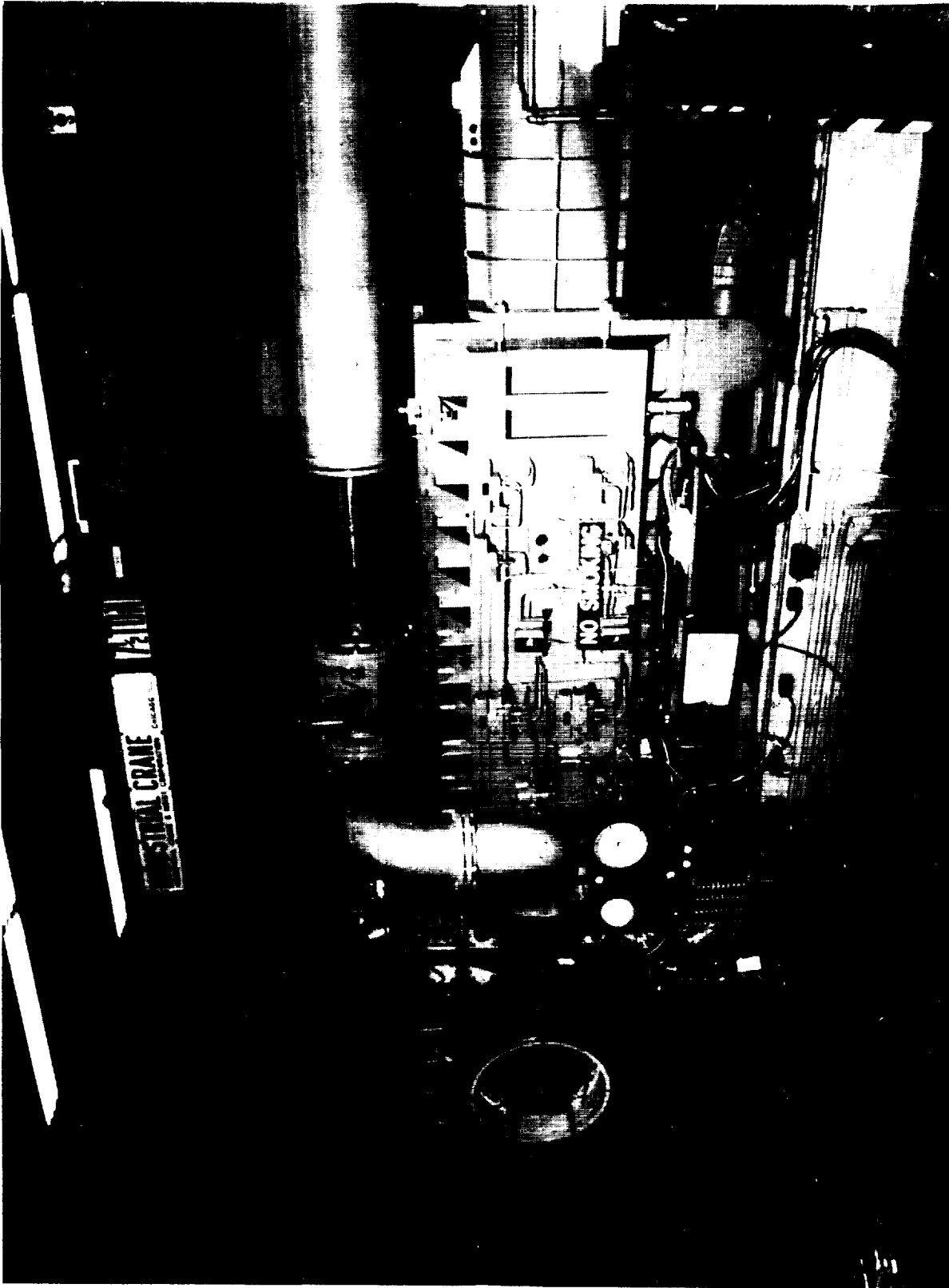
Figure 1. MSFC's 14-x14-inch trisonic wind tunnel facility.
