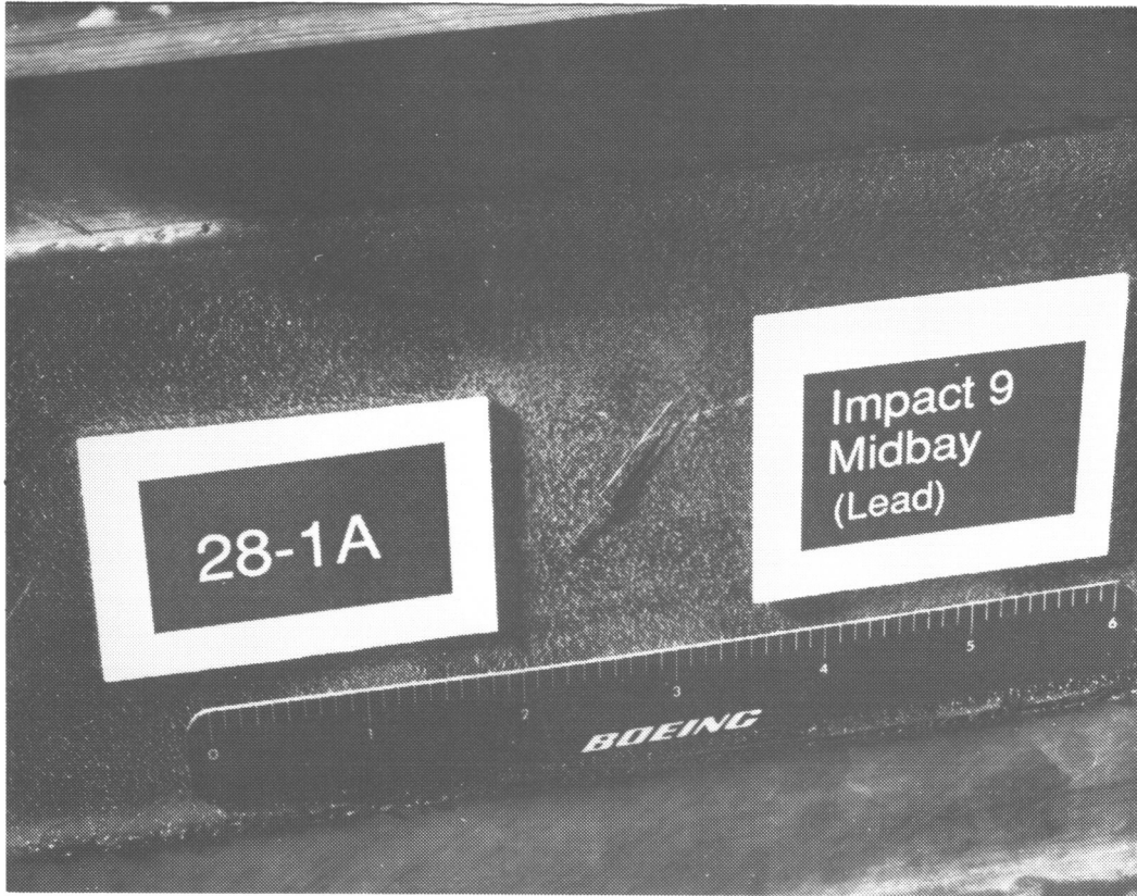
Figure 14: Barely Visible Damage.
