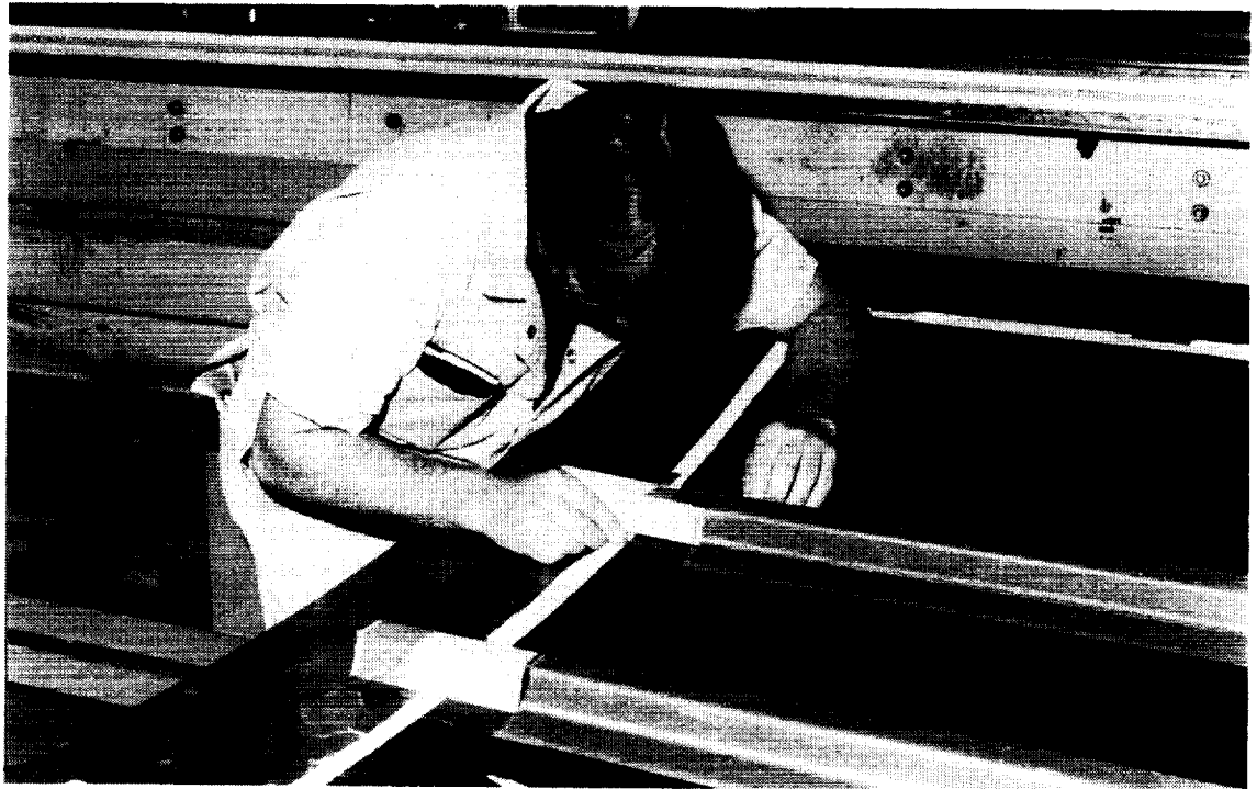
Figure 15. During assembly, stringers were located to the skin IML using a straight edge to ensure precise location.
