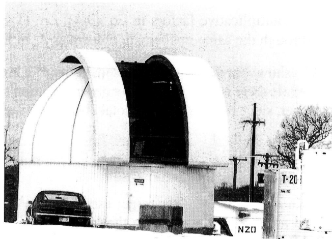
Figure 9-3. Photograph of the CW laser remote sensing observatory at the Goddard Optical Research Facility.
