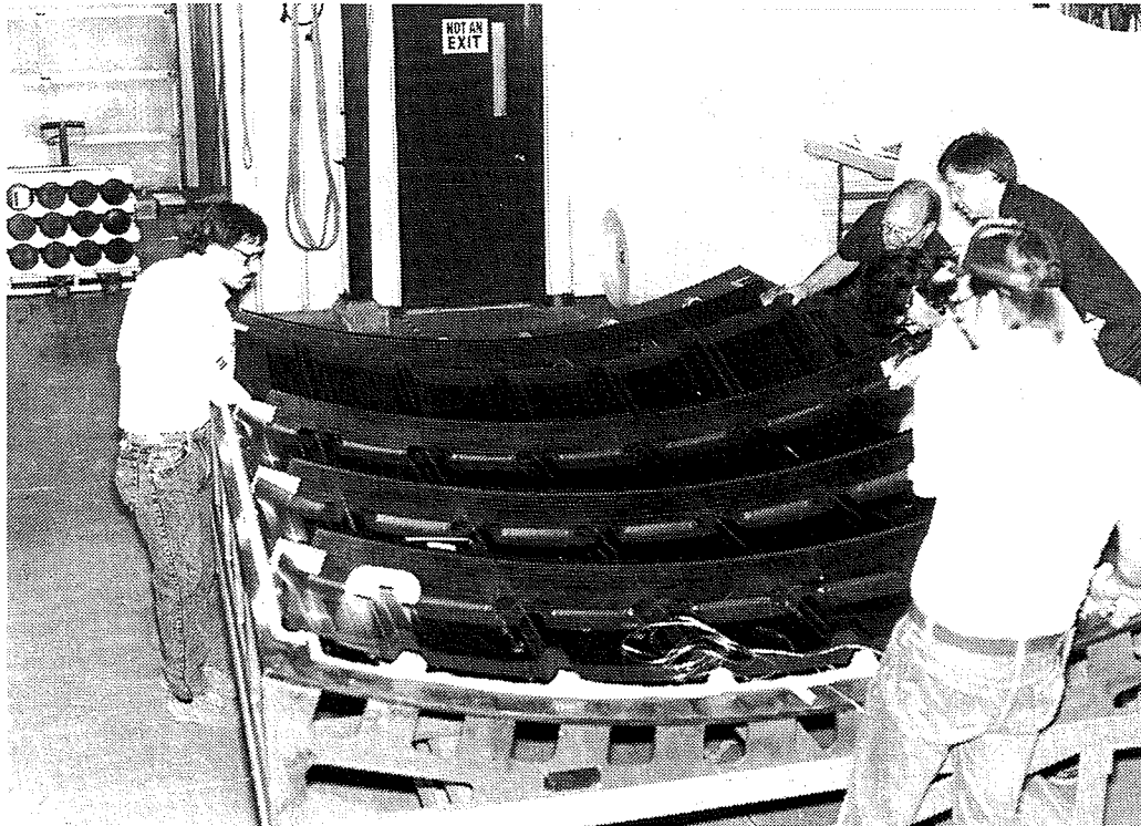
Figure 3-50. Installation of Cauls
