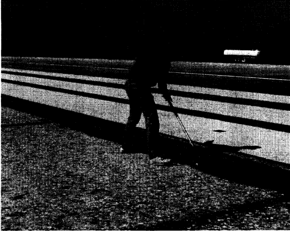
(a) Application to corduroy surface.
