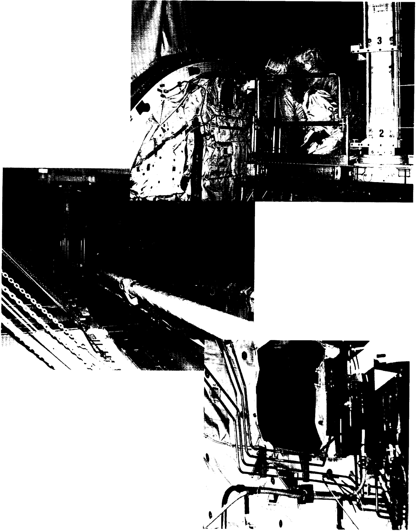
1/4-Inch Cooling Plate Tube Ultrasonic Flowmeter Test on Discovery
