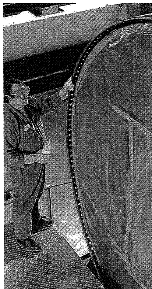
Figure 13. Handcleaning During Nozzle Installation
