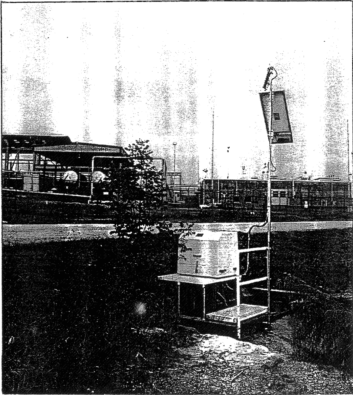
Figure 4. Solar Powered Remote Monitoring Site; LMTAS Outfall 3
