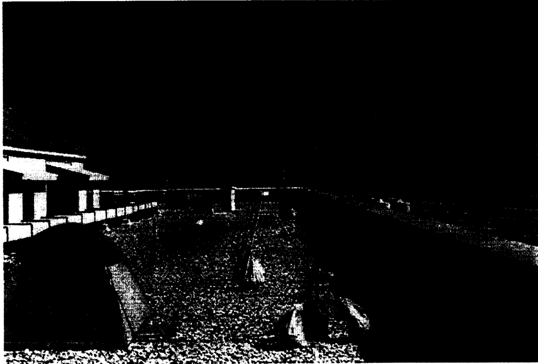
Figure 2 Stouffer's Hotel Antenna Installation
