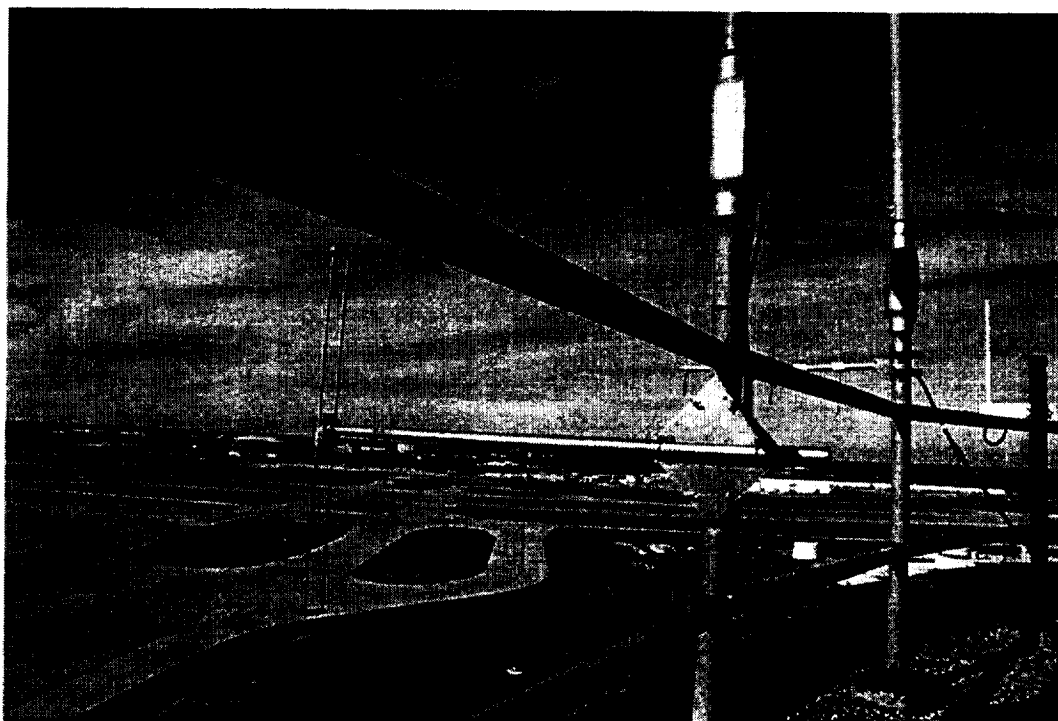
Figure 1 Control Tower Antenna Installation
