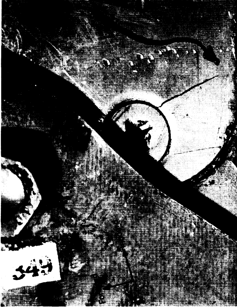
L-59-179 Figure 12.- Crack in left trailing-edge skin just aft of hole 401. Photograph made at low-gust maximum, spectrum 9.
