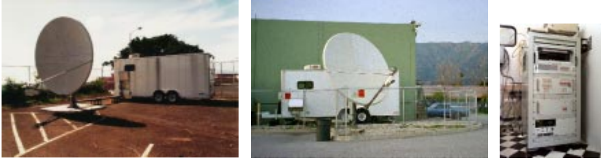
Figure 1: The ACTS high data rate (HDR) ground stations: a. The HDR at Tripler Army Medical Center in Honolulu, Hawaii. Visible are the 12-foot antenna and associated equipment trailer, connected by a dry waveguide. Note the very low elevation of the antenna, due to the extreme western longitude of Hawaii. This low elevation exacerbated rain fade problems. b. The HDR at JPL in Pasadena, California. c. The control unit inside each HDR equipment trailer. From top to bottom, the rack contains a real-time Unix control system with SONET I/O boards, a burst modem, and a high-output transmitter.
