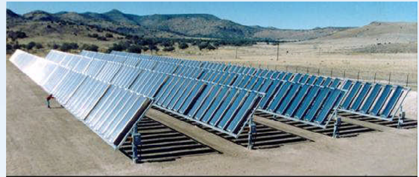
100 kW Terrestrial Array with Si Cells (TX)
