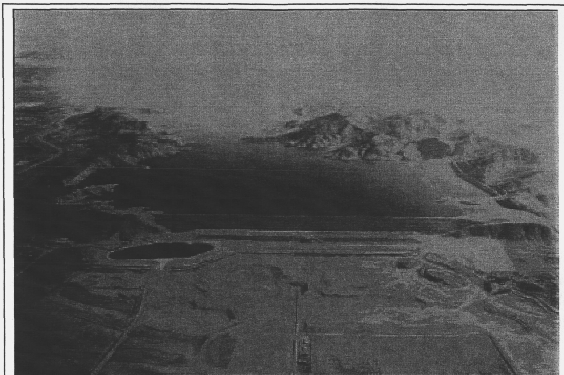
Figure 8. MWD's Diamond Valley Lake. This reservoir contains a 6-month emergency water supply for southern California, and lies between two active geologic faults (San Jacinto and Elsinore). There are 9 1 Hz GPS stations monitoring three earthen dams.
